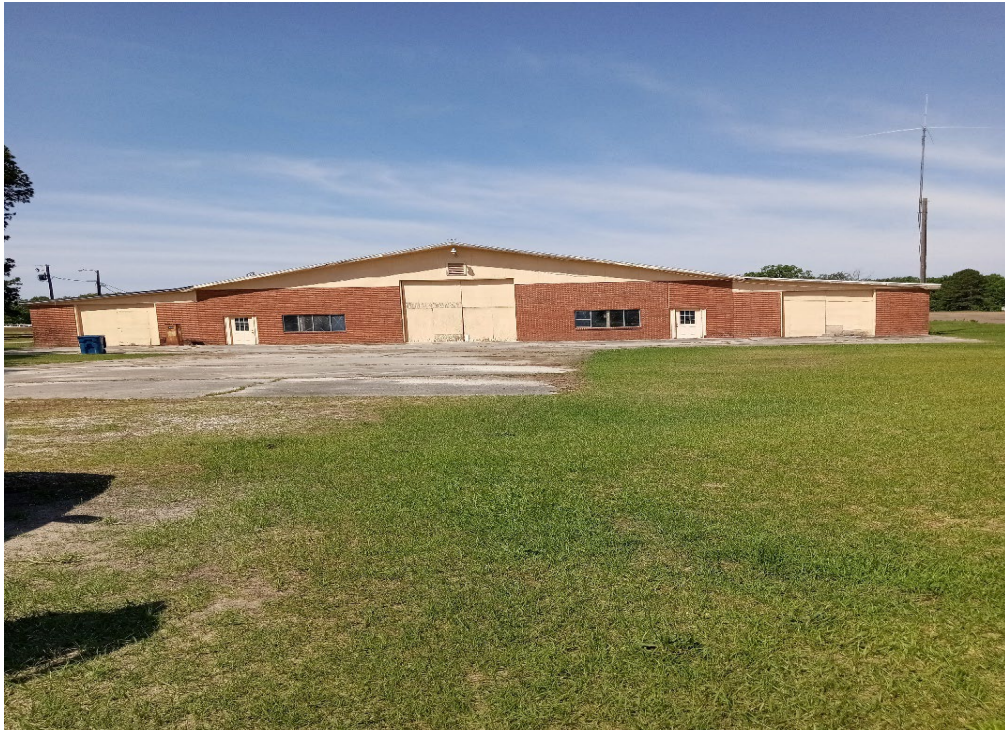
Existing Warehouse located on the property.
