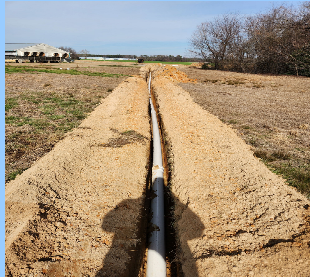
Underground Irrigation installation on a swine farm
