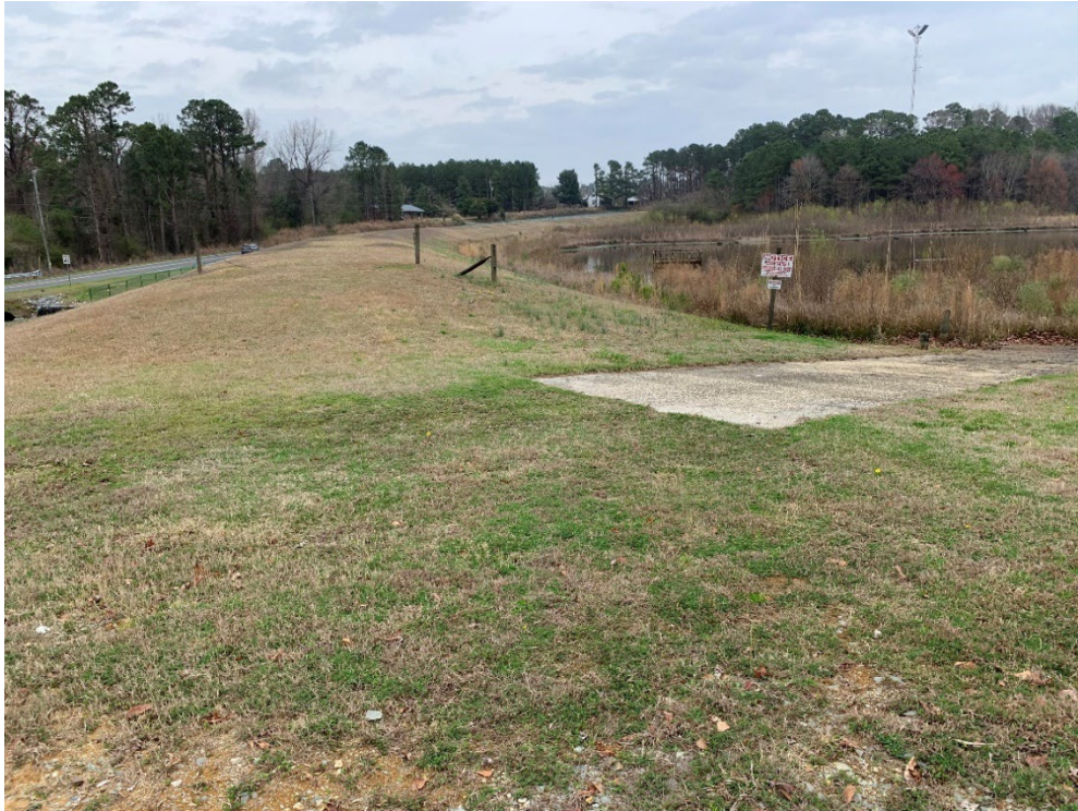
Photo 1 – Dam Access / Top of Dam
