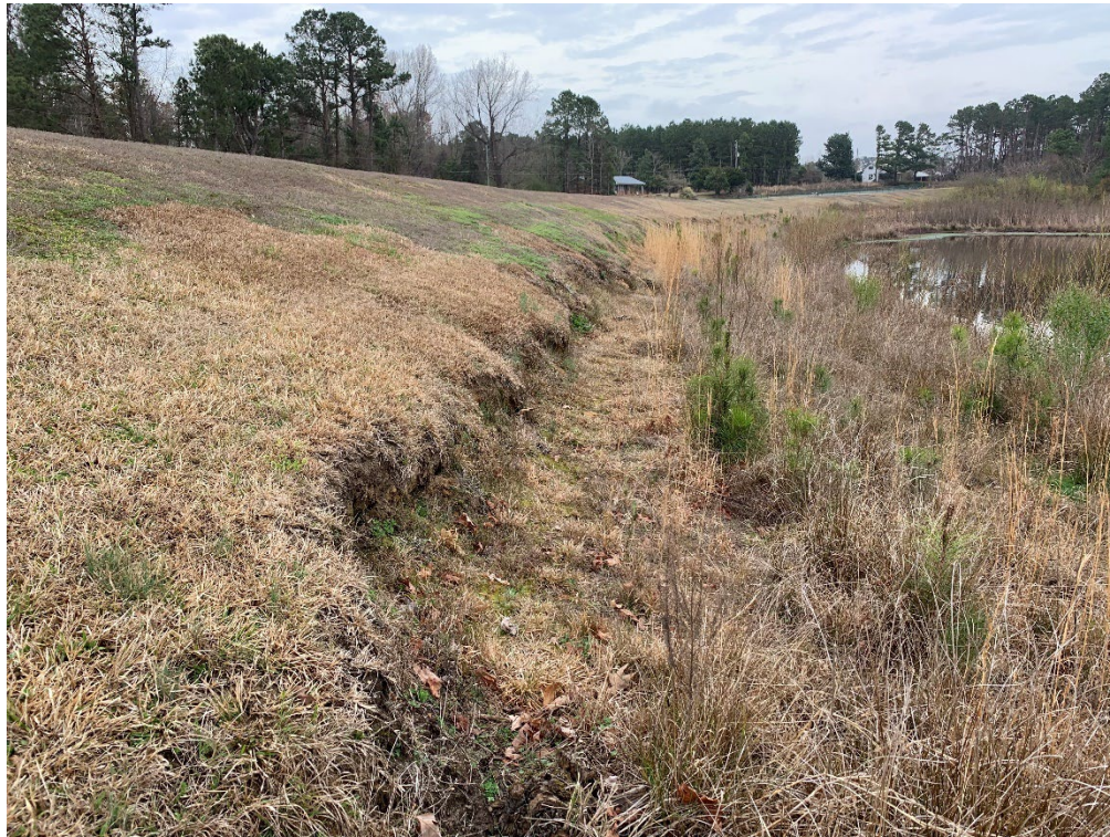
Photo 3 – Upstream Slope of Dam
