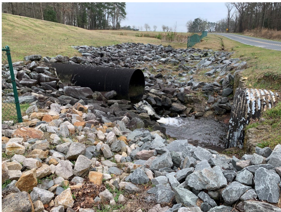
Photo 6 – Primary Spillway Outlet
