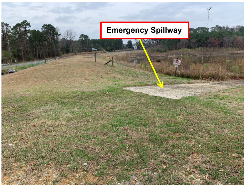
Photo 4 – Top of Dam
