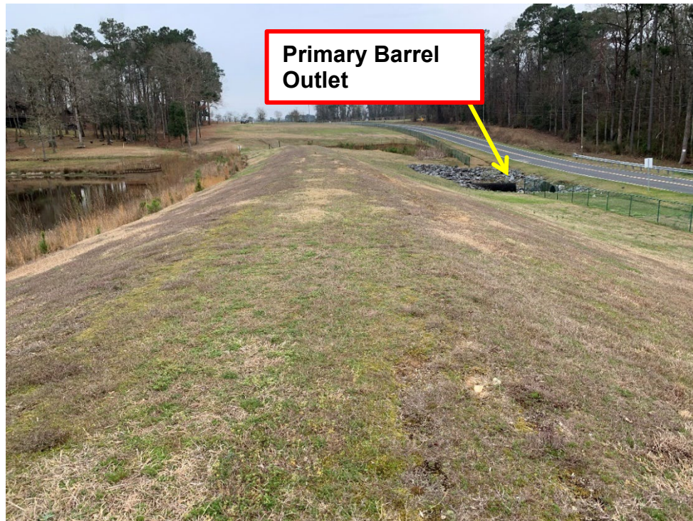
Photo 5 – Top of Dam
