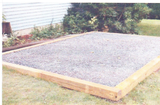
Similar Crush n' Run Pad. The barriers we build will be 3 sided. (20x20x30 ft.)
