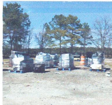
Current Electronics Recycling Area- No Designated Area
